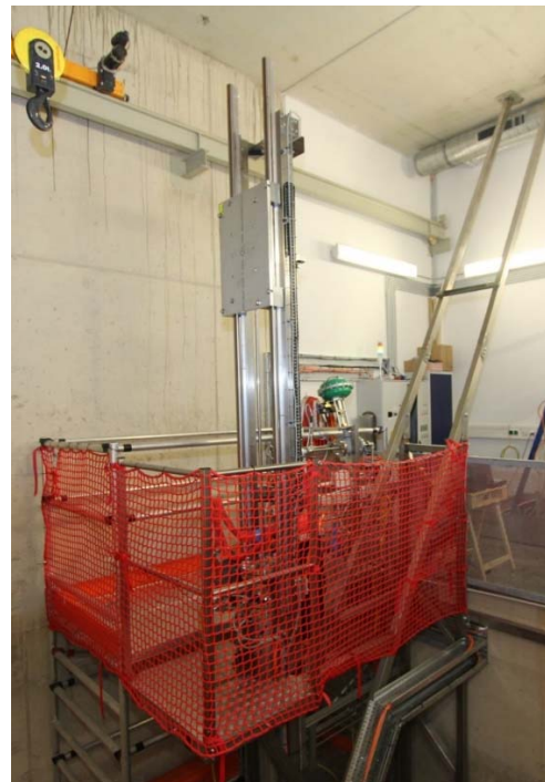
Figure 8: Pump Testing Facility
