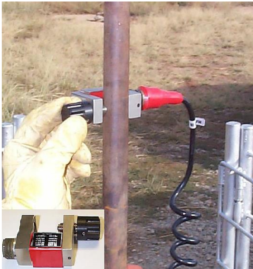
Figure 14: Installation of a PRT dynamometer (Downhole Diagnostic, 2020)
