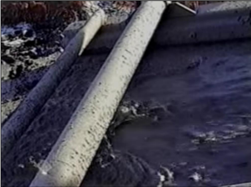
Figure 10: Mud Overflow After Addition of the Fibrous Material to Suspend Cuttings and Clean the Well (Forta Corporation 1997)
