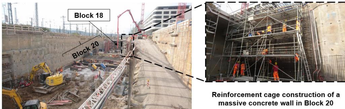
Fig. 67: On-site photos replicating the construction process of Block 20
