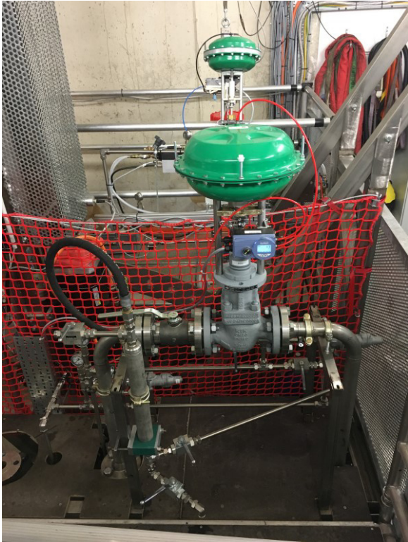
Figure 61: Pneumatic regulating valve and sampling device
