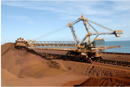
Fig. 3. Photograph of the reclaimer from which the data for Table 2 were acquired.
