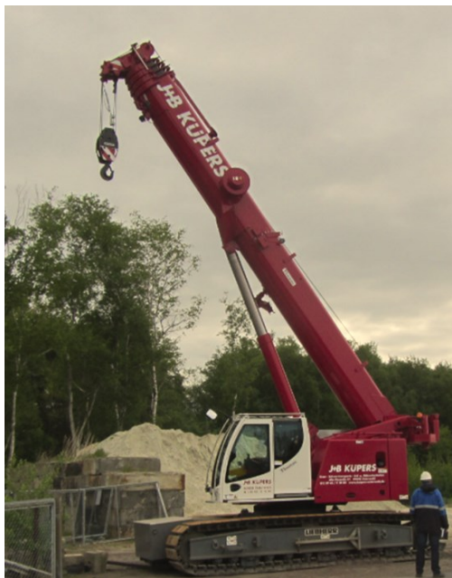
Figure 3.19: 60 t crawler crane
