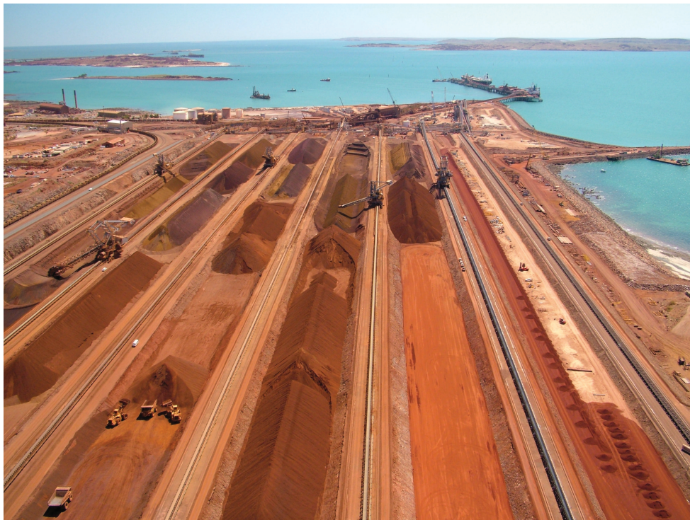
Figure 2.4: Longitudinal stockyard (courtesy of Sandvik)
