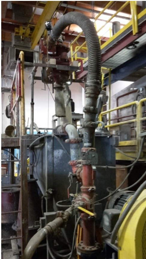
Figure 21: Test rig from the view of the pump
