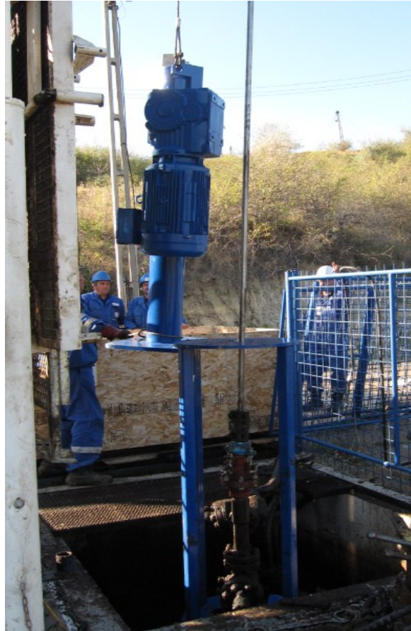
Figure 15: Installation of LRP in Moldova Sud
