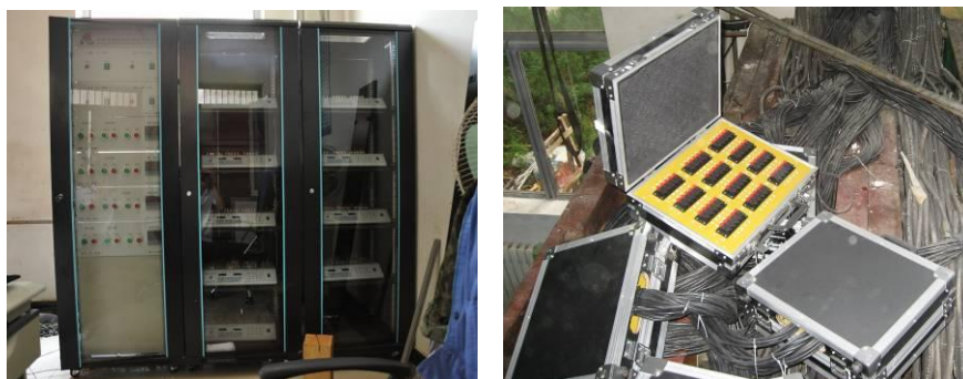
Fig.3.3 Data collection system
