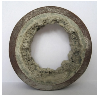
Figure 55: Scale deposit in a pipe
