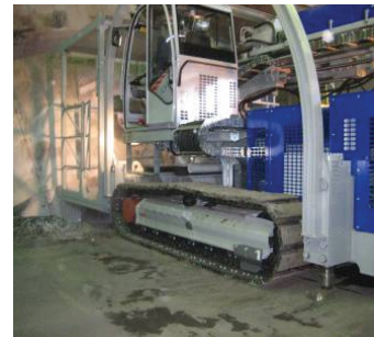
fig. 71: positioning of TBD and calibration of the floor pots
