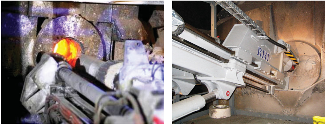
fig. 46: inserting new taphole
