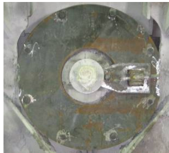
fig. 70: installation of retaining mechanism
