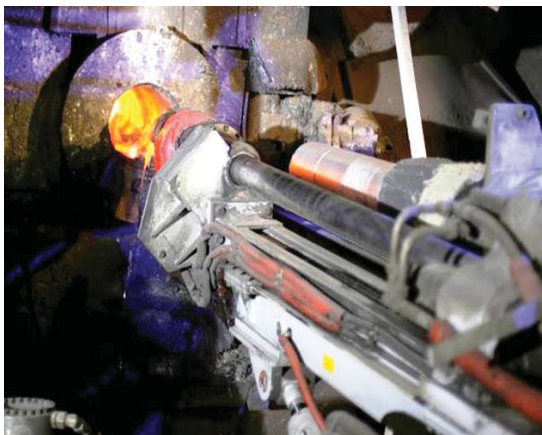
fig. 45: backwrecking of the worn taphole and cleaning of taphole channel
