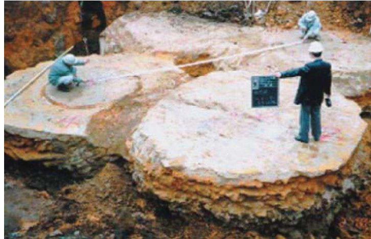
Figure 214 Picture of a jet grouted body [33]
