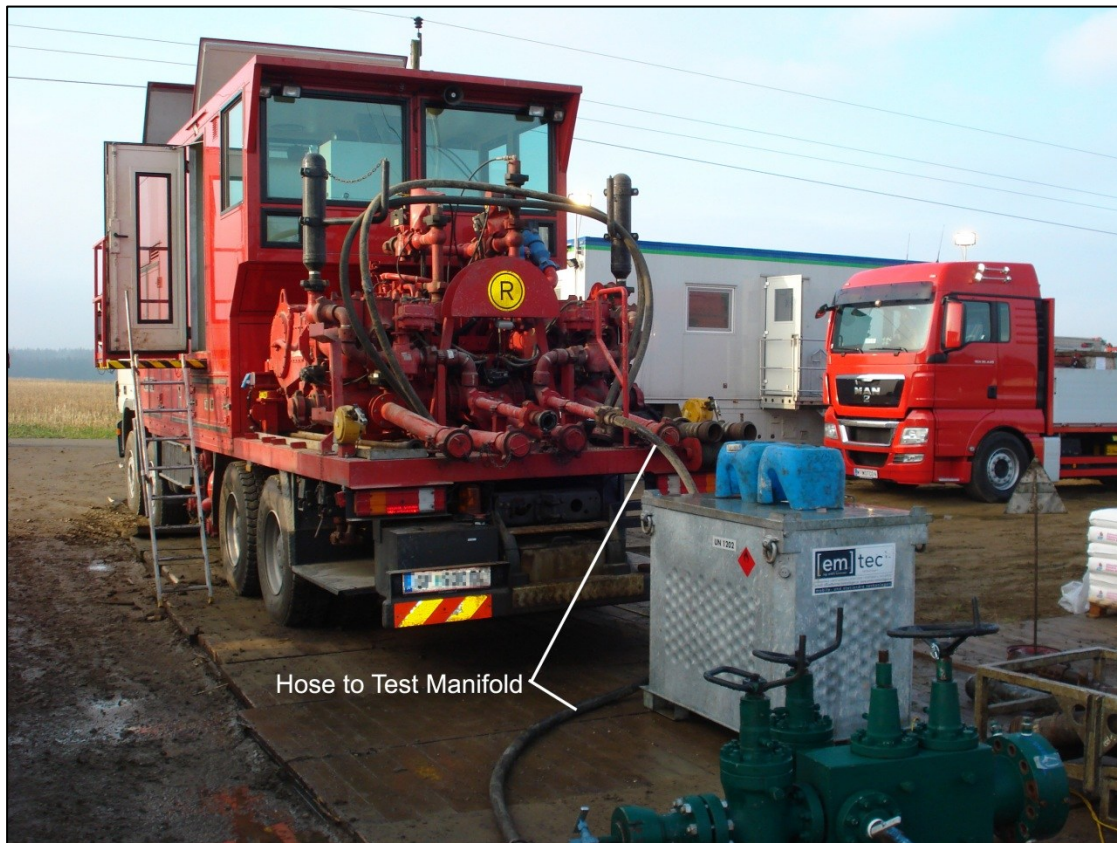
Figure 10 – OMV Cementing Unit during an Extended Leak-Off Test
