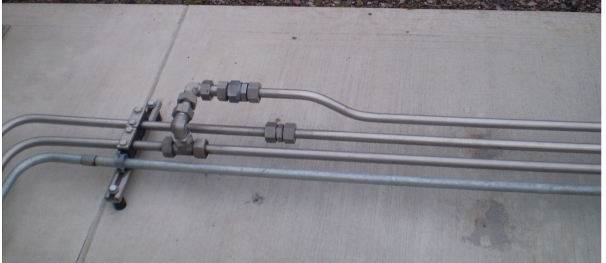
Figure 15: Bypass for the hydraulic pressure line [1]
