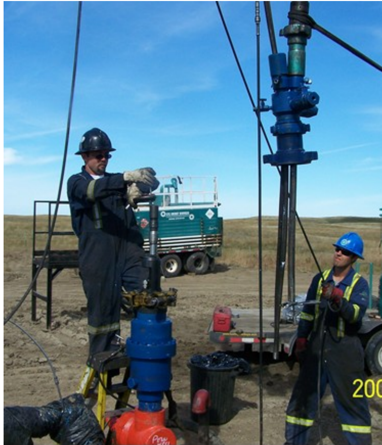
Figure 41: Installation of the Tri-Coil Wellhead [50]
