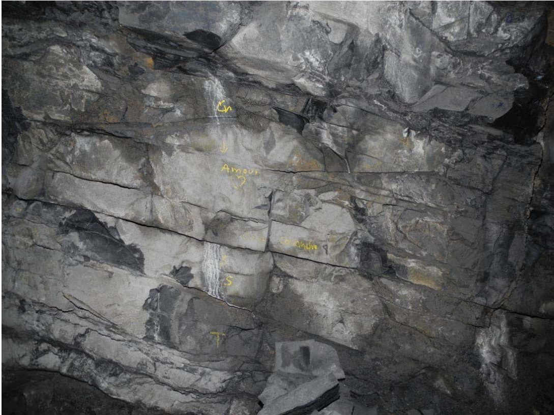
Figure 12: Layer Cr – T, connection passage (east wall)
