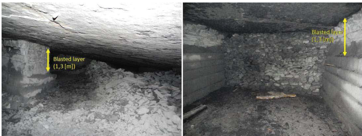
Figure 34: Examples of backfill
