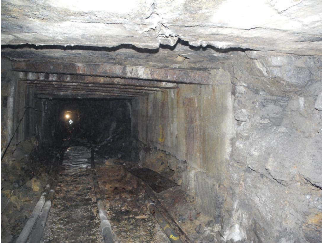
Figure 15: Support major fault „17m“, connection passage
