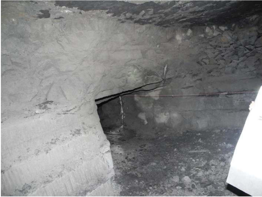
Figure 23: Major fault „inside“; photo number: 1760
