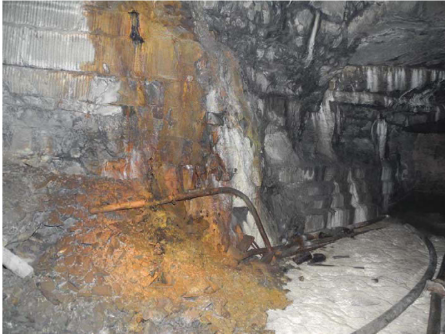
Figure 25: Major fault „inside“; photo number: 1464
