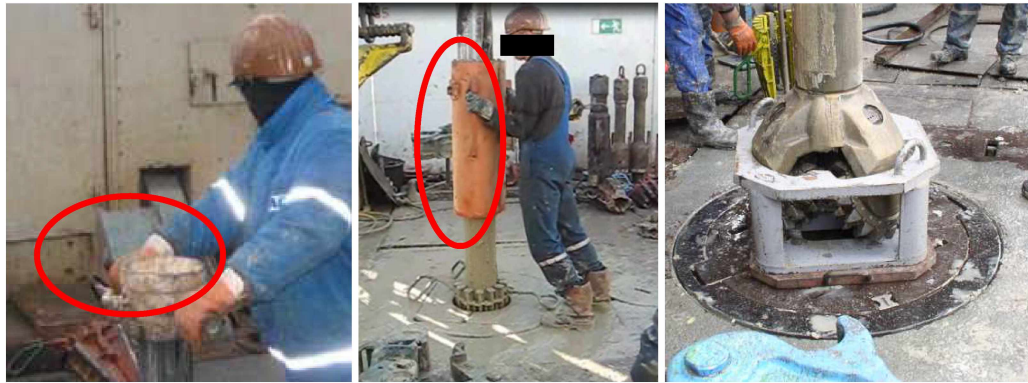
Figure 25: Step-in guide (left), mud bucket (middle), bit breaker plate (left)
