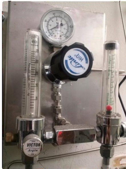
Figure 65: Control valves for the nitrogen flow and pressure adjustment
