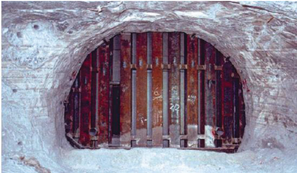
Figure 47: Fill barricades in lower level of the mine 29 p.37
