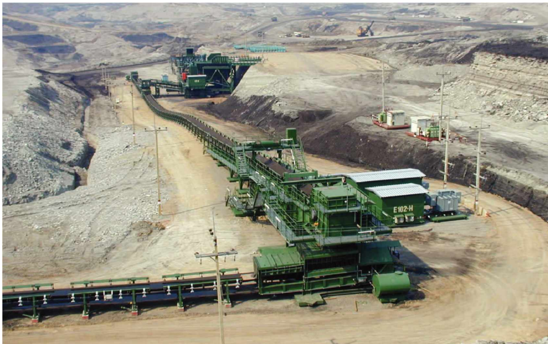
Fig. 3-37: Belt conveyor system VABCS 1800 in mine
