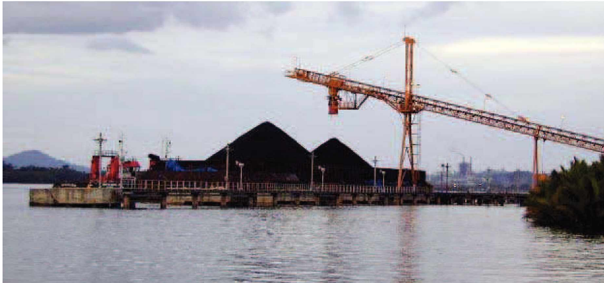
Fig. 3-31: Spreader with 2 separate stockpiles
