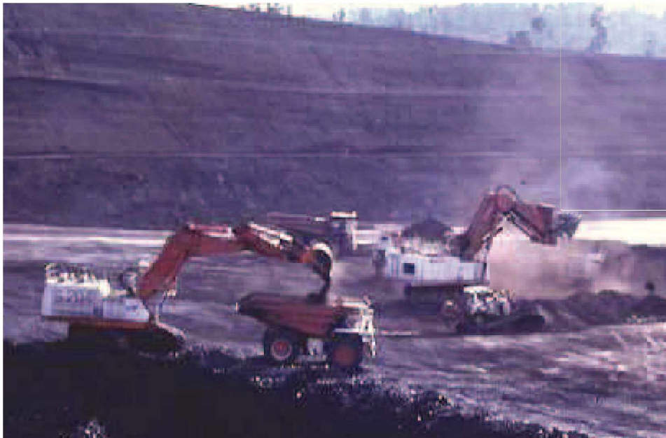
Fig. 3–29: Hydraulic shovel excavators Liebherr Type R996 loading trucks in the pit
