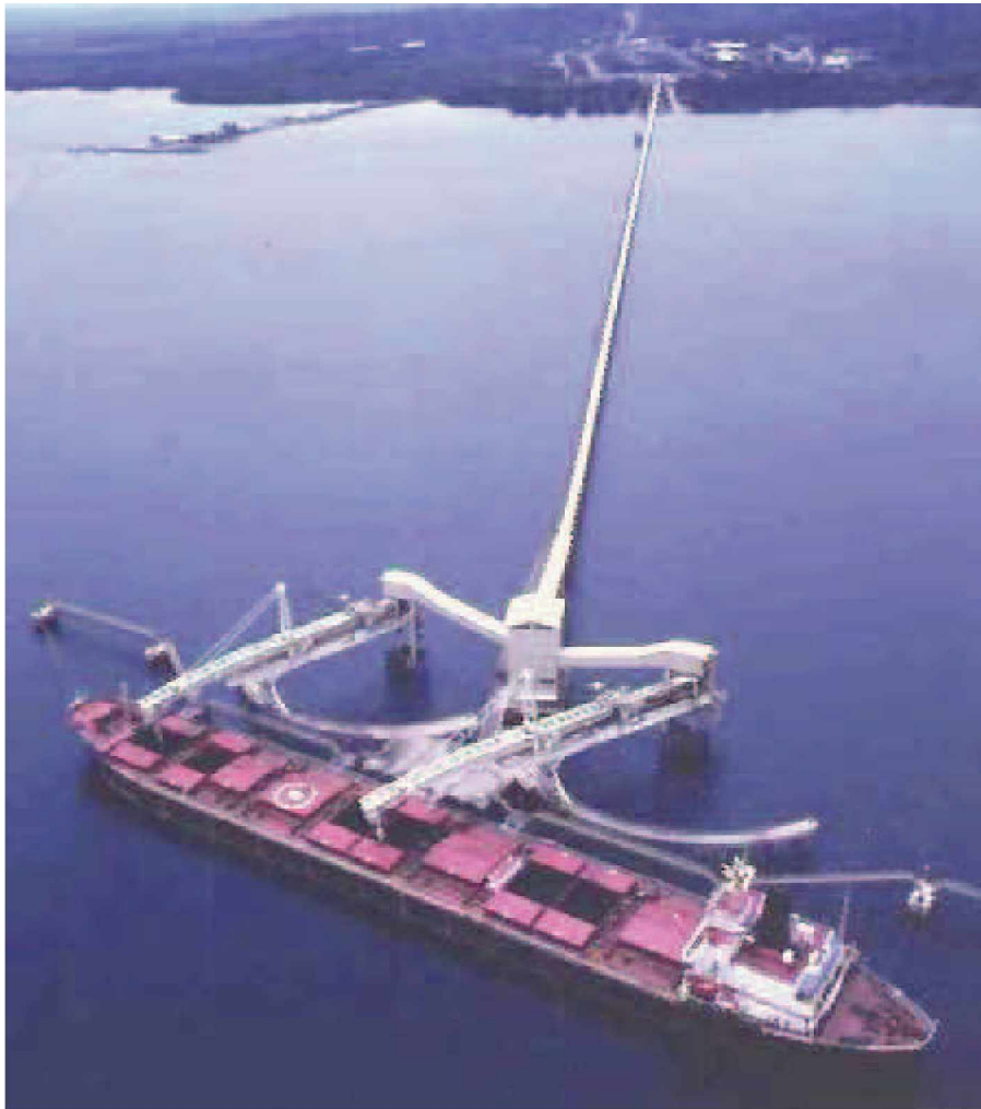
Fig. 3-32: Overland conveyor for ship onloading
