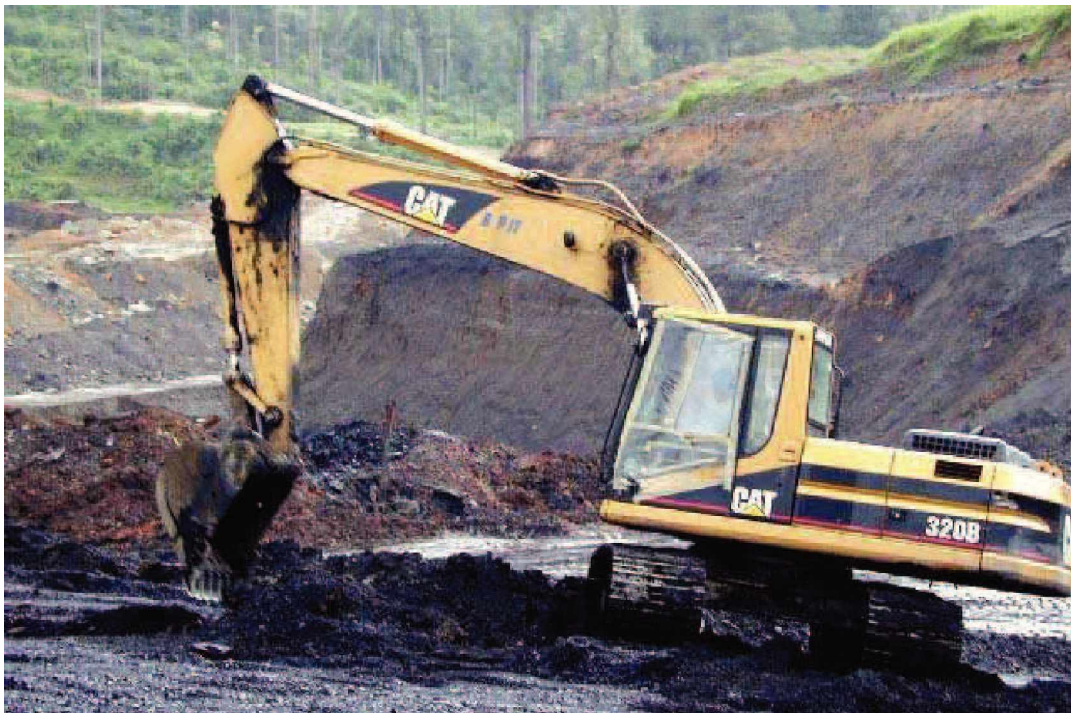
Fig. 3–28: Hydraulic shovel excavator Caterpillar Type 320B
