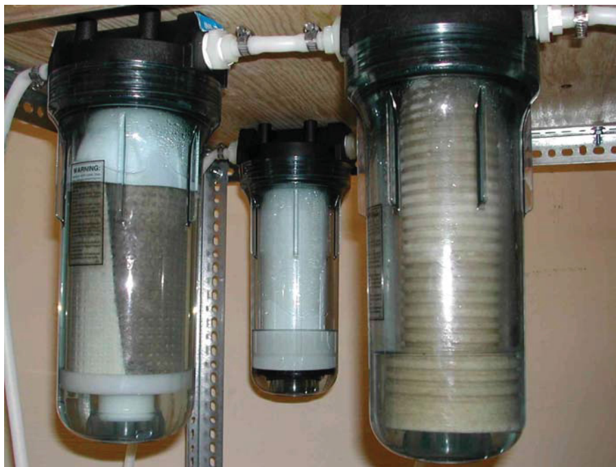
Figure 3.7: Pretreatment unit, close-up
