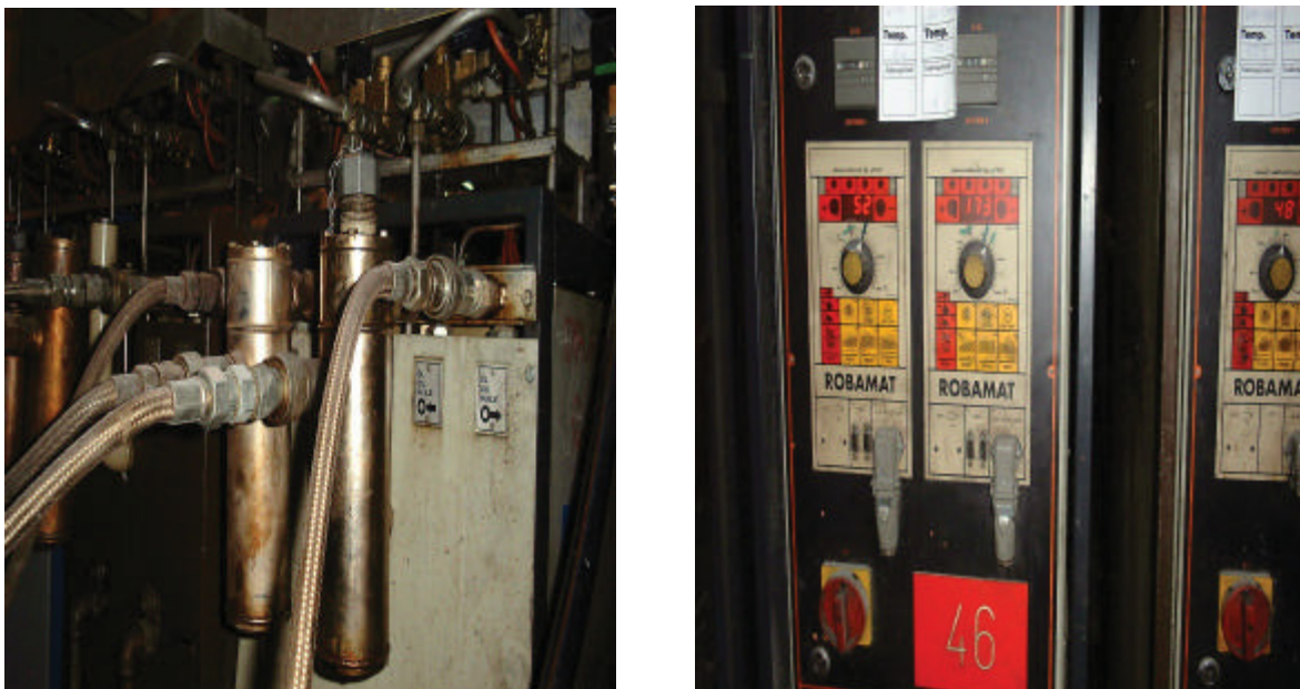
Diagram 2.3.2.1: The ROBAMAT heat exchangers during operation (l = back view, r =front view).
