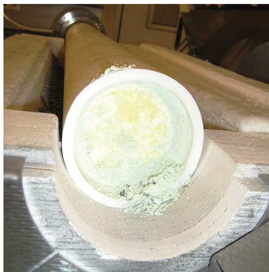
(b) Broken pipe with blockage within the kiln at the end of the heating zone "D-Mo 2"
