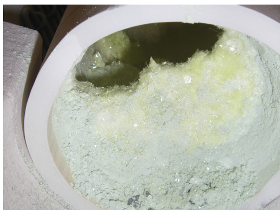
(c) Broken pipe with blockage within the kiln at the end of the heating zone "D-Mo 2"
