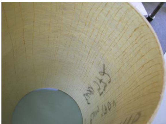
Fig. 3.4: Pipe segment with cracks
