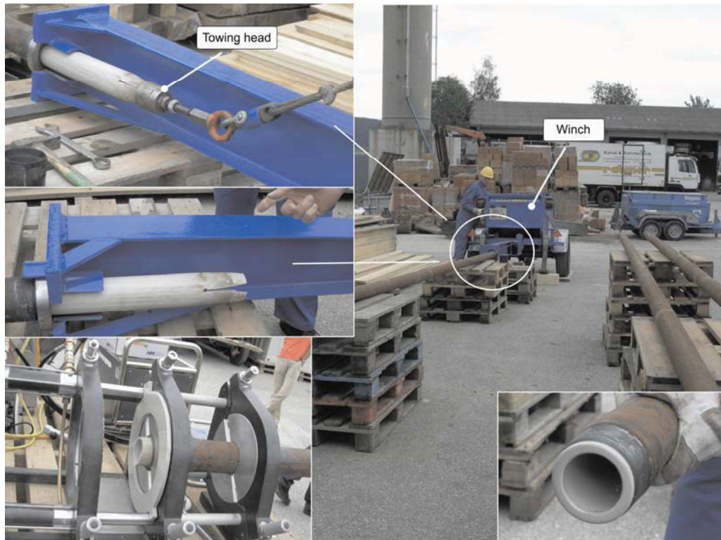
Figure 2.8: Relining process for OMV AG.
