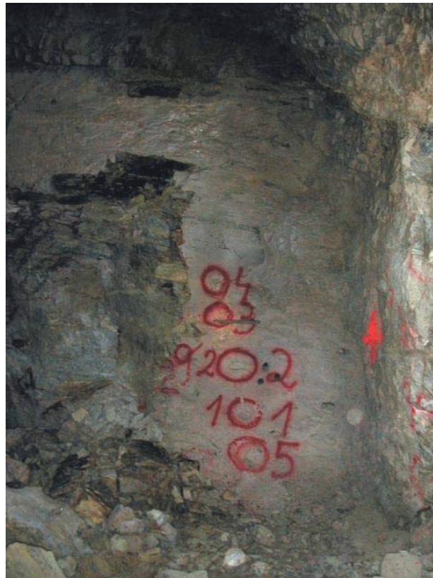
Figure 6.10: Arrangement of the boreholes in the sidewall, test area University of Leoben at the Erzberg Iron Ore Mine
