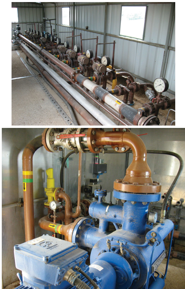
Figure 54: Multiphase pump of RAG in Zistersdorf
