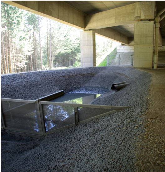
Figure 15: The infiltration basin under the bridge 45 (SLP 02, 03, 04, 05)
