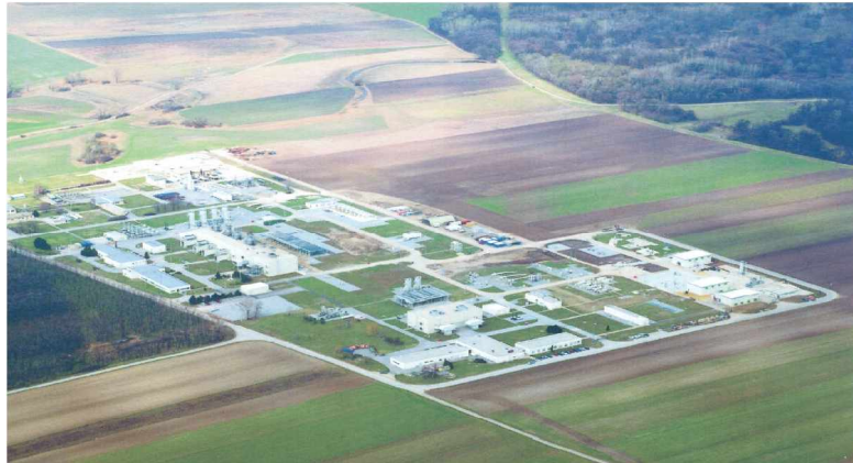
Figure 19: Compressor station in Baumgarten
