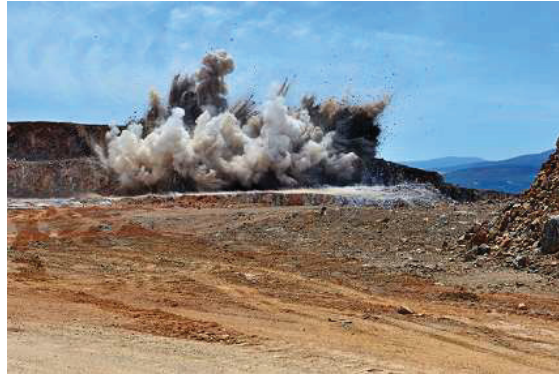
Figure 2-2 Rock blasting ( www.mining-technology.com )
