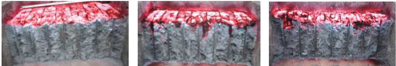
Figure 3-15 Alpha block surfaces after blasting of 1st, 2nd and 3rd rows
