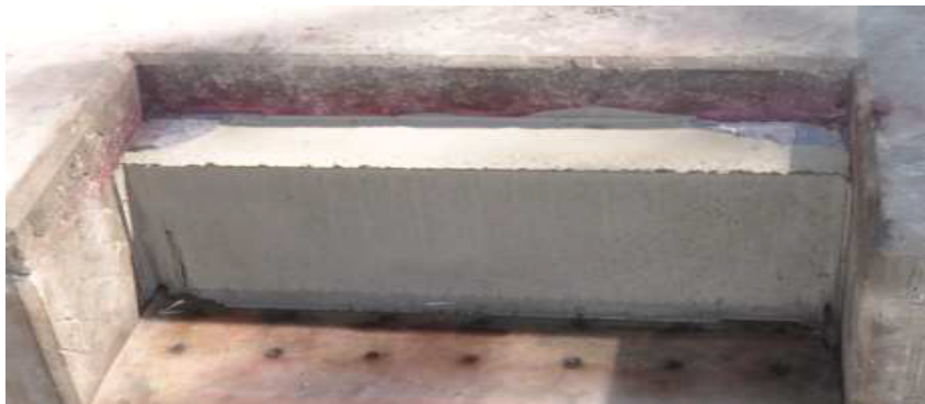
Figure 3-18 JS3 Alpha after fast hardening cement was poured.
