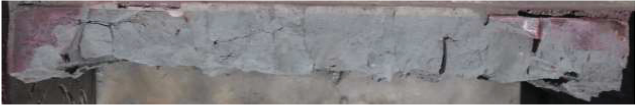
Figure II-4 JS1 Alpha top view after blasting of 3 rd row
