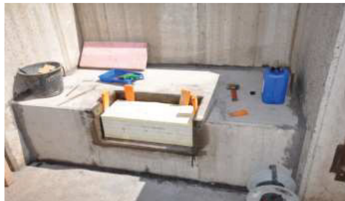
Figure 3-3 Block installation and test specimens and procedure
