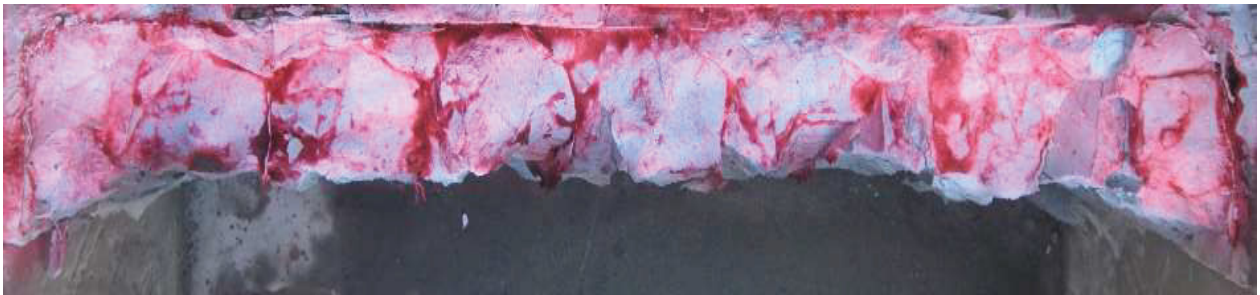
Figure II-70 JS4 Beta top view after blasting of 3 rd row
