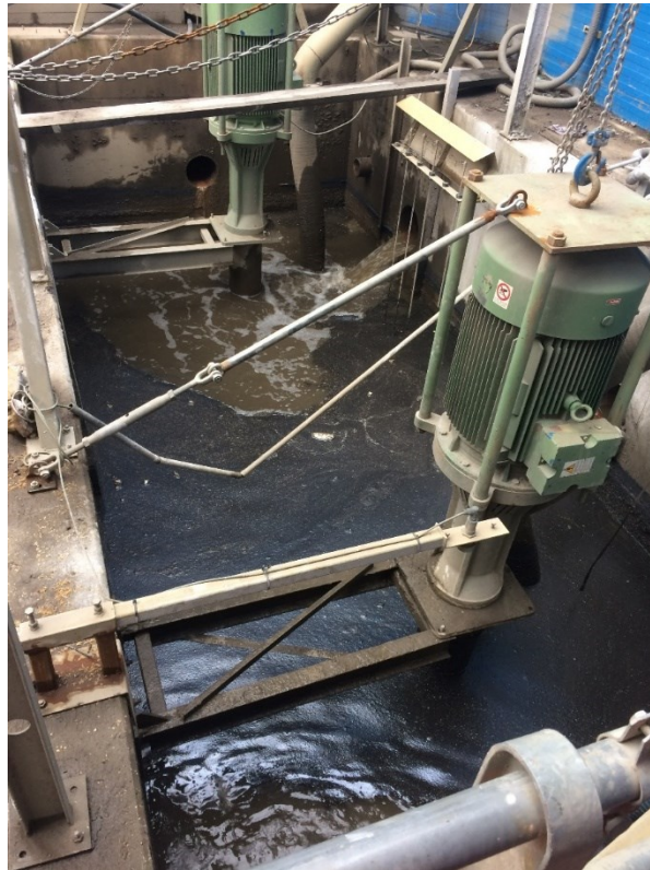
Figure 28: The united pump sump, already without concrete wall
