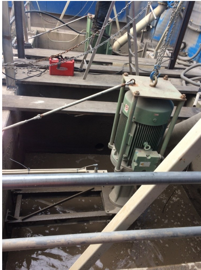
Figure 26: Right pump sump with a view on the separation wall
