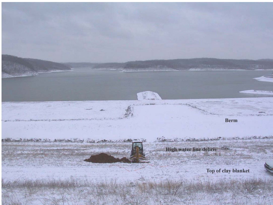
Figure 3-1. Sinkhole in dam formed from piping of dam fill through karst features in bedrock. Backhoe digging out sinkhole in Clearwater Dam, Missouri, USA, to follow throat that was significantly deeper than machine can dig (photo by S. Hartung).
