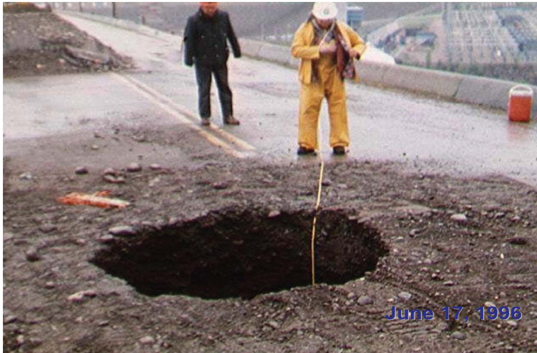
Figure 4-12. Sinkhole with throat extending tens of meters into fill material over impervious core in Bennett Dam, British Columbia, Canada (photo from website). Sinkhole in dam formed from piping of dam fill through karst features in bedrock.
