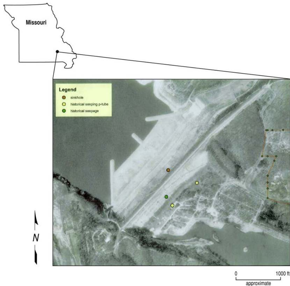
Figure 1: Aerial photo of Clearwater Dam. Sinkhole and seepage are indicated. Dikes extending into the lake were part of the 1989 retrofitting for seismic stability and seepage control.
