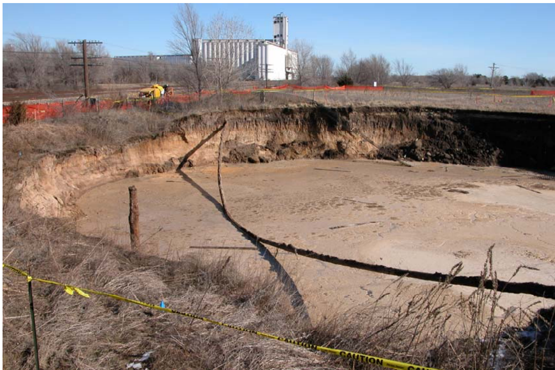
Figure 1-7. Mosaic sinkhole 12 days after catastrophic collapse on January 7, 2005. Obvious in this photograph is solution mining well #19 (left side of sinkhole), an unused gas pipeline suspended across the sink, and a heavily used set of railroad tracks fewer than 25 m north of the sinkhole edge (photo by R. Miller).
