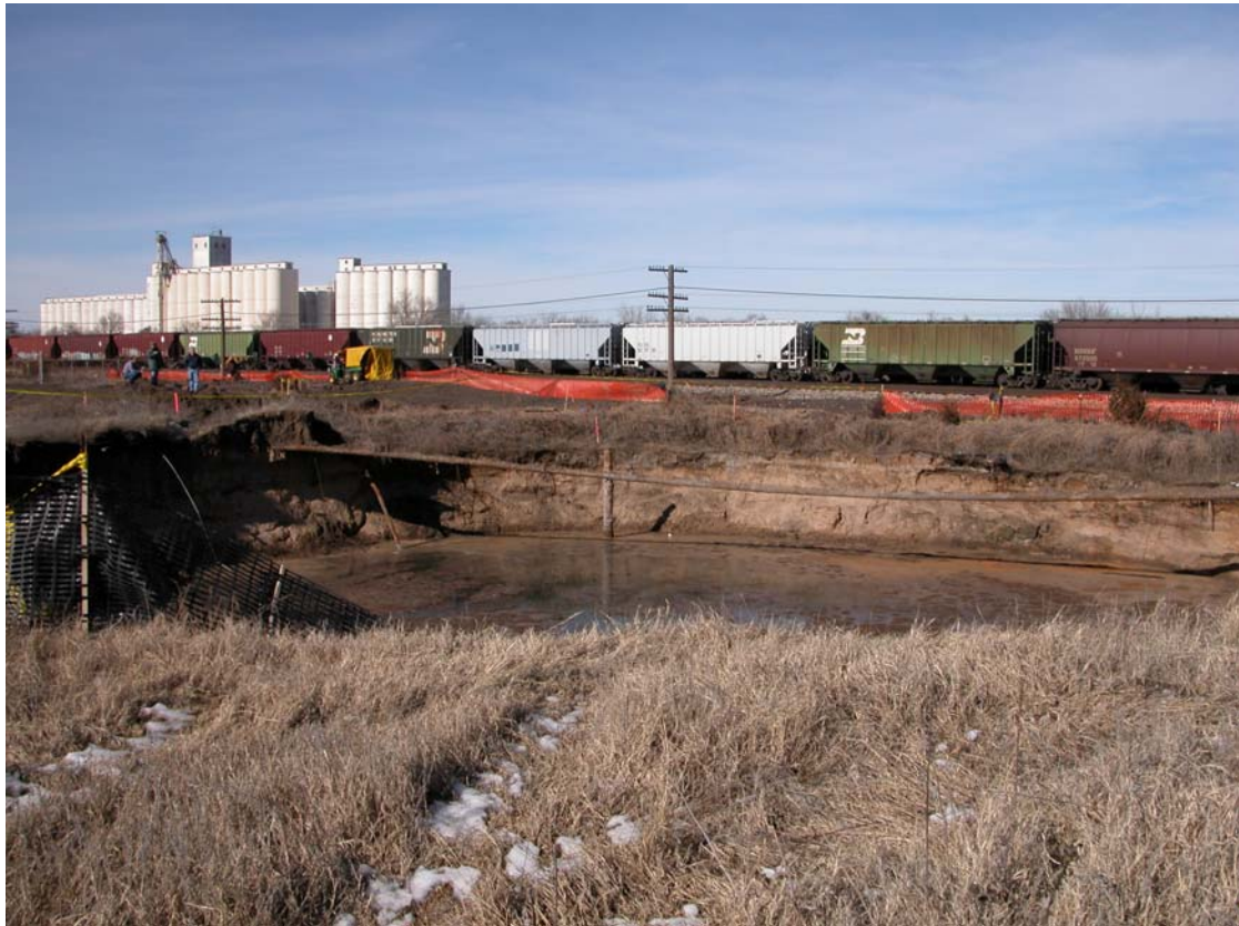
Figure 9-18. Mosaic sinkhole growing radially at about 1 m/day 12 days after catastrophic collapse on January 7, 2005. Obvious in this photograph is solution-mining well #19 (center of photo), an unused gas pipeline suspended across the sink, and a heavily used set of railroad tracks fewer than 25 m north of the sinkhole edge. Also pictured is the seismic crew and recording vehicle (yellow cover) (photo by R. Miller).
