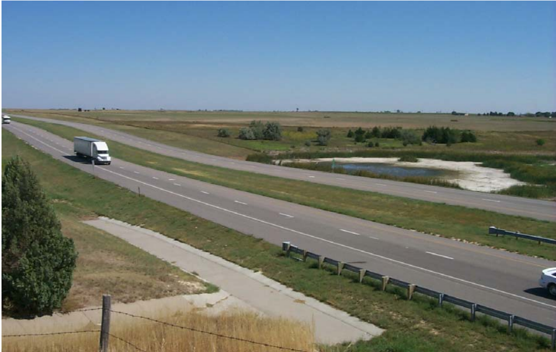
Figure 1-4. A stretch of Interstate 70 between Russell and Hays, Kansas, began subsiding in 1967, one year after the highway was opened. Surface subsidence has been consistent and gradual at about 20 cm/year for almost 40 years (photo by R. Miller).
