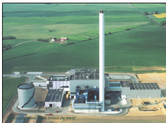
Figure XVI.5: Straw power plant - European reference photos [ETV, 2006]
