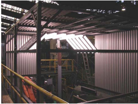
(a) Housing under construction
