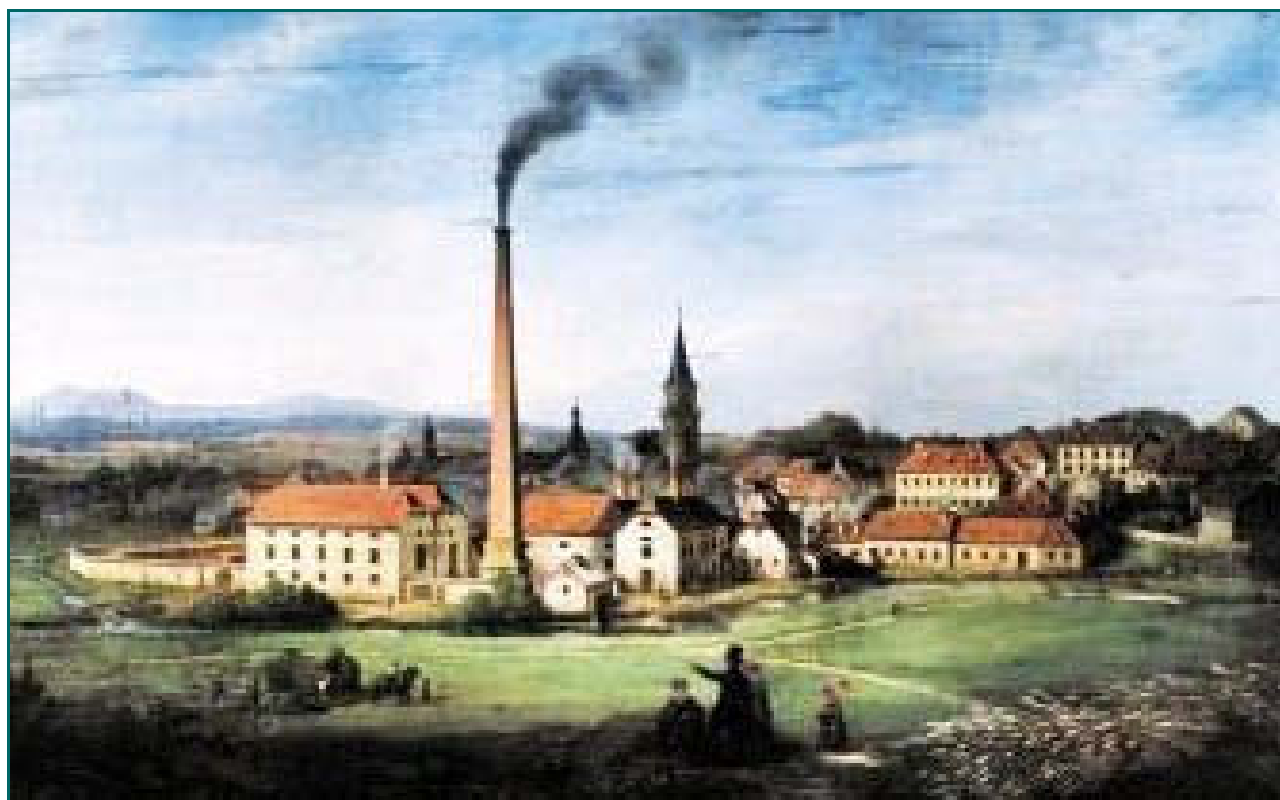
Figure 4-27: View of the Chemical Factory Marktredwitz in 1860 after an oil painting from a contemporary unknown artist (Marktredwitz, city archive)
