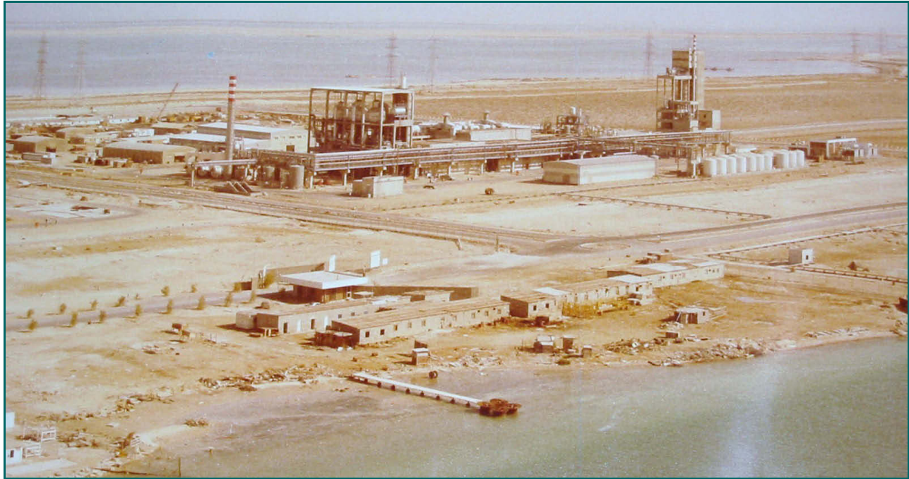
Figure 1-1: Chlorine-alkali electrolysis plant in the Middle East (Site remediation supervised by the author in 2004/05)
