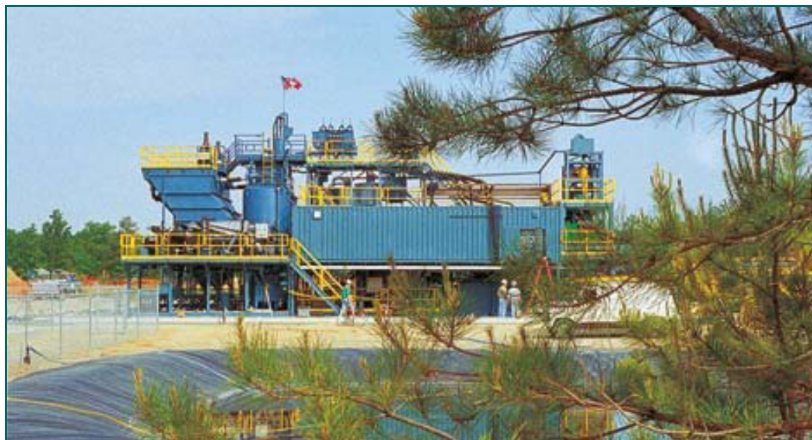
Figure 5-8: Soil washing plant for the King of Prussia (KOP) Superfund site in New Jersey (Source: Metso Minerals)
