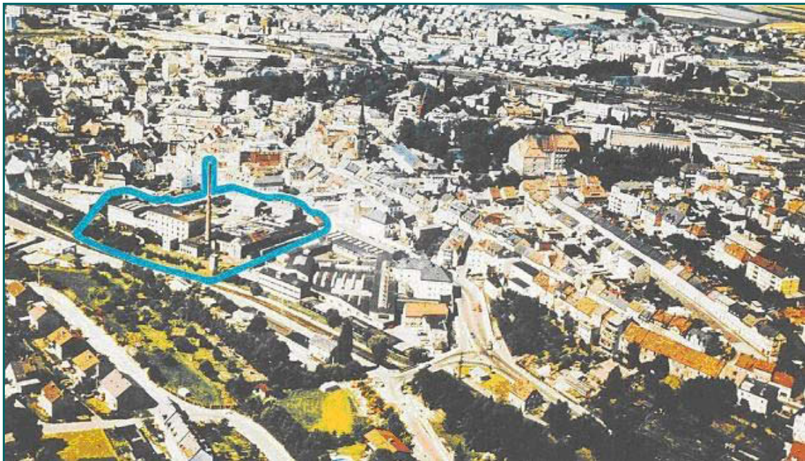
The Chemical Factory Marktredwitz was the first large-scale mercury remediation project worldwide (photo: Harbauer)
