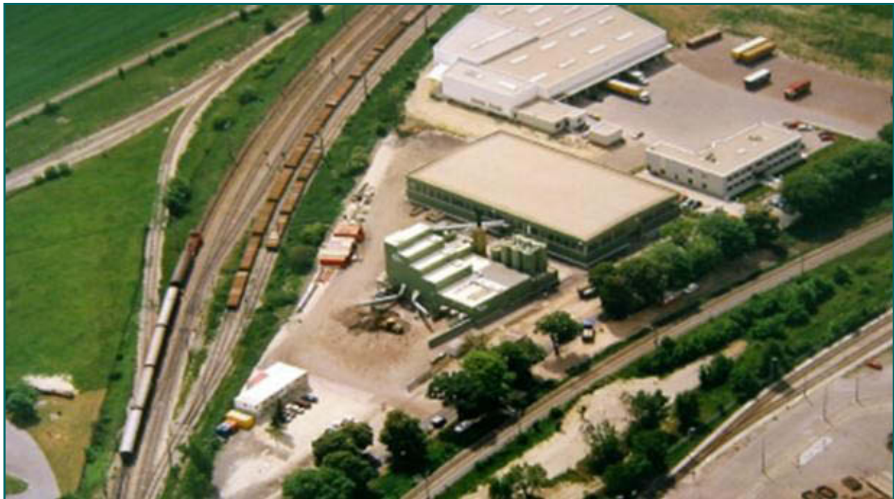
Figure 5-3: Bird's view of the physico-chemical soil processing plant in the 11th city district of Vienna (Source: ABW)
