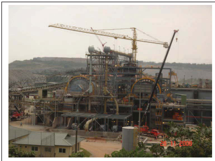
Figure 93: Tarkwa Gold, expansion 2008. On the left side the original plant and on the right side extension plant with new mill, pumps and cyclones, picture Roman van Ommen, 2009
