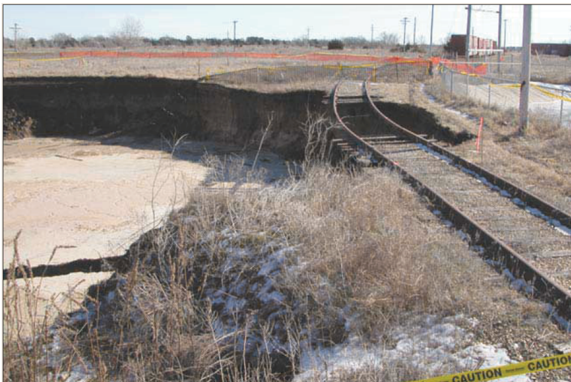
Figure 5.1 Sudden formation of a sinkhole within the city of Hutchinson near an important railroad, in 2005 (from Lambrecht et al, 2006).
