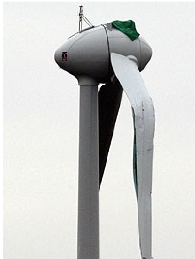
Figure 1.6: Fatigue failure of a composite rotor blade in Conisholme, Lincolnshire, 2009 [23].
