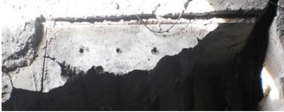
Figure 90: Extensive back breakage damage (B5R1, free face) (Petropoulos, 2011)
