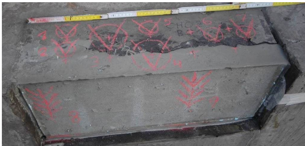
Figure 67: Space after blasting filled with fast hardening cement
