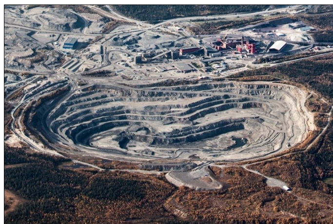
Figure 2. Former Leveäniemi open pit after it has been emptied of water in 2014 (Photo: LKAB).
