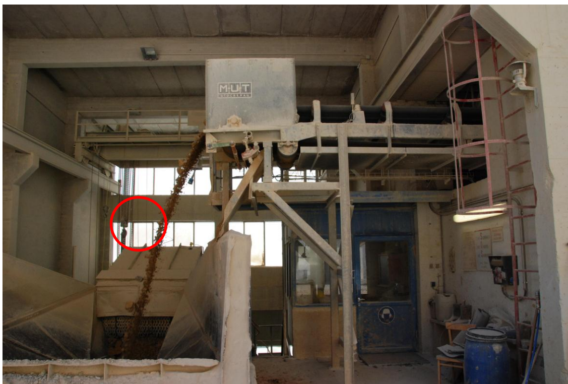
Figure 13: Transfer point belt conveyor - crusher
